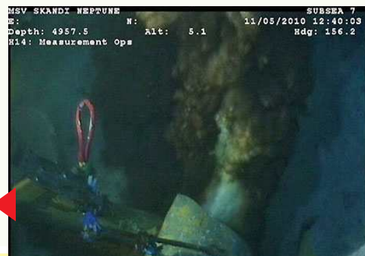
Picture of oil gushing from the riser pipe on the sea floor almost 5000 feet down below the Gulf of Mexico
